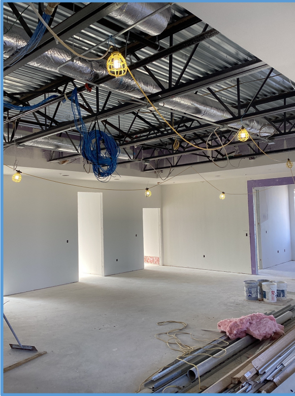
Interior 2 nd Floor Open Office Area 11/07/23
